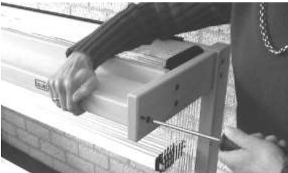
Fasten the shelf front to the top side pieces, using two of the 50 mm screws.
