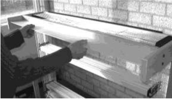
Slip the shelf bottom into the slot of the front rail. You may need to loosen the screws at the side pieces one turn.
